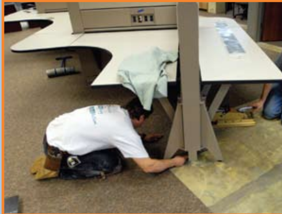
The new carpet is slipped under the partitions.
