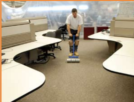
Roll the new carpet to ensure adhesion and we are done!
