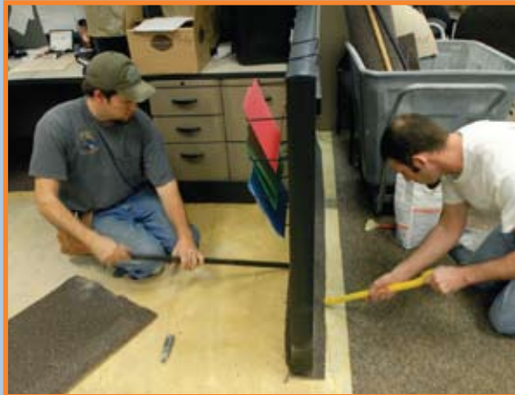
We gently pry up the partitions to facilitate old carpet removal.
