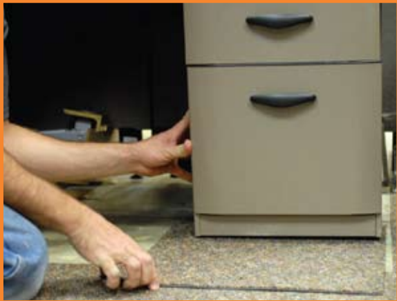
While lifted, we slide new carpet tile under the equipment.
