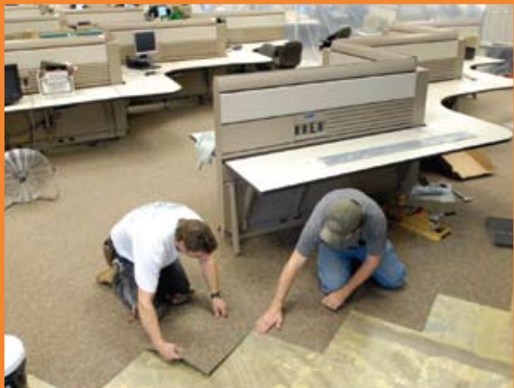
The field carpet is installed.
